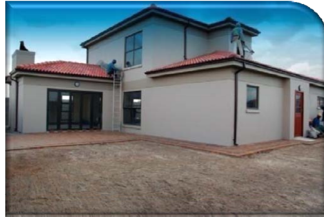
Steel frame residence
