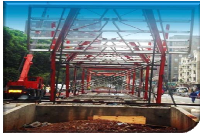
Steel structures for BRT
