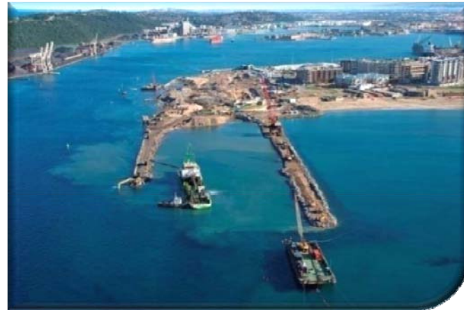
Widening & deepening Durban harbour
