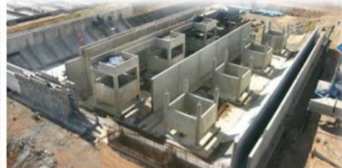
Themba Water Treatment Works South Africa In progress
