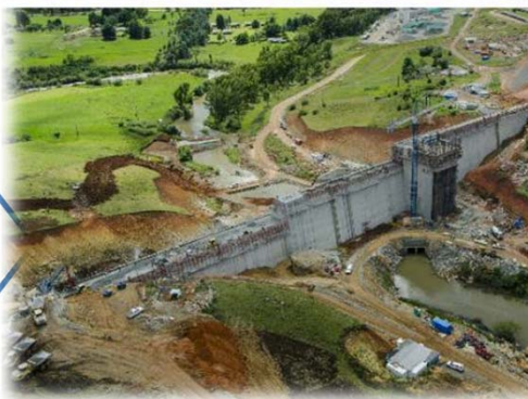
Spring Grove Dam South Africa Complete Water from the dam will be transferred from the Mooi River catchment to the Umgeni River catchment to augment water supplies (by 60 million m3/annum)
