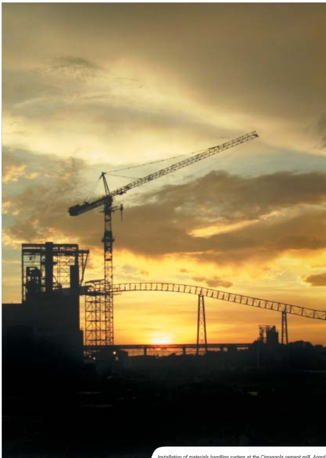
Installation of materials handling system at the Cimangola cement mill, Angola
