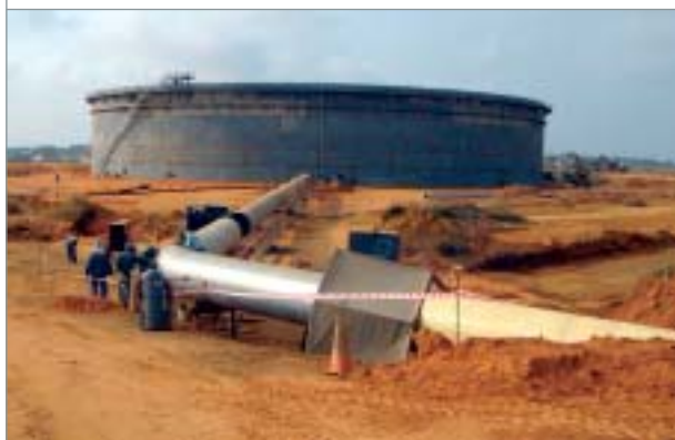
Tank 11 at Cabinda, Angola, involved the group's multi-disciplinary expertise
