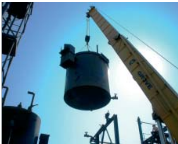
Moving an entire copper processing plant from O'kiep in the North Western Cape to Ruashi in the DRC involved several heavy lifts
