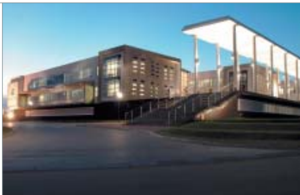
New premises for the Building and Housing operations in Woodmead, Gauteng
