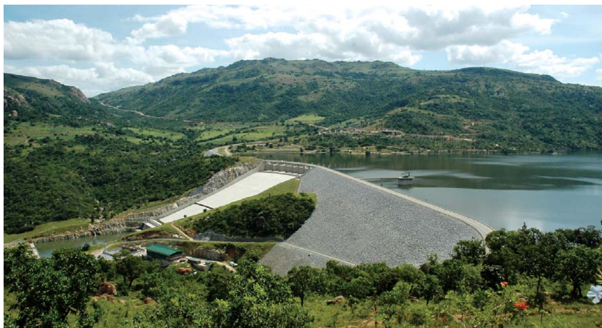
Strict environmental regulations were observed during the construction of the Maguga hydro power station
