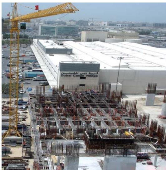
Construction on the Mega Cargo terminal at Dubai International Airport
