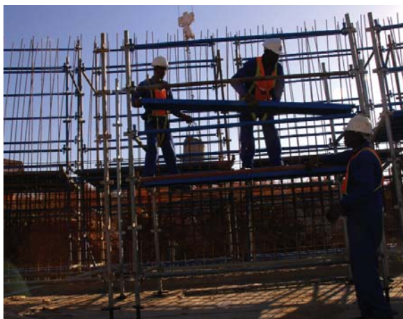
Workers at the Sunderland Ridge waste water treatment plant, Centurion
