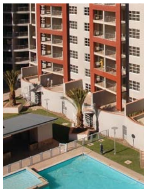
Sandhurst Towers in Sandton comprises two multi-storey apartment blocks
