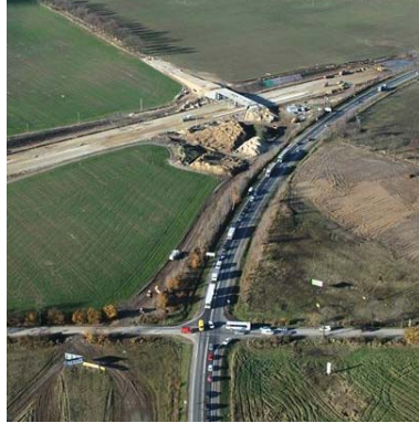
Construction on the A1 freeway in Poland. The concession achieved financial close in July 2005
