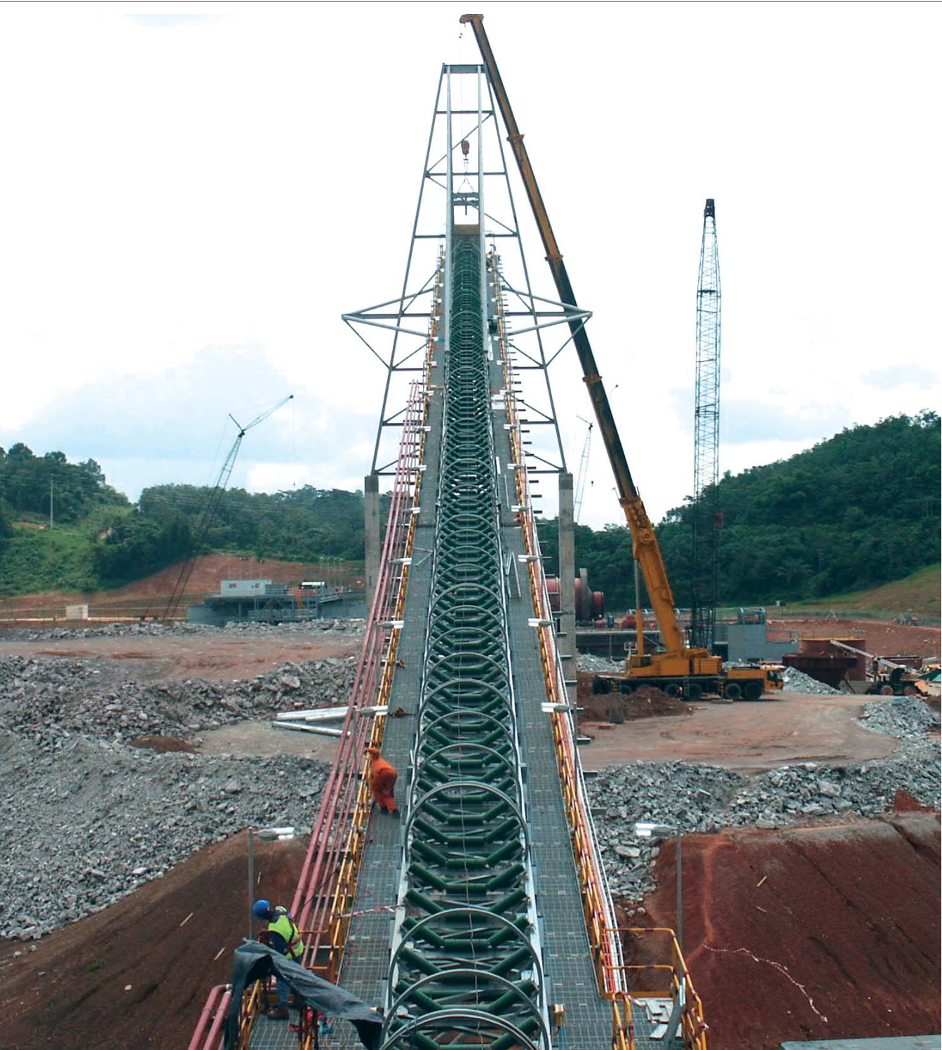
Installation of a conveyor system at Tarkwa gold mine in Ghana
