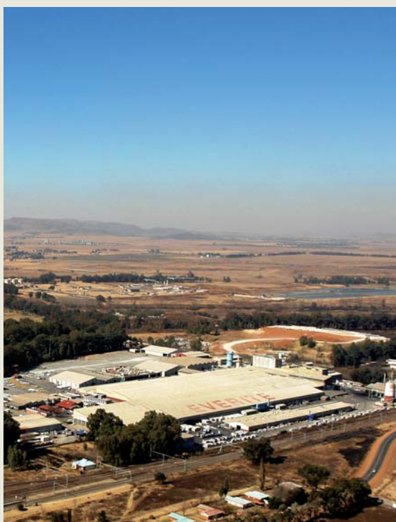
The Everite dump site is being covered with a view to closing it by the end of 2007
