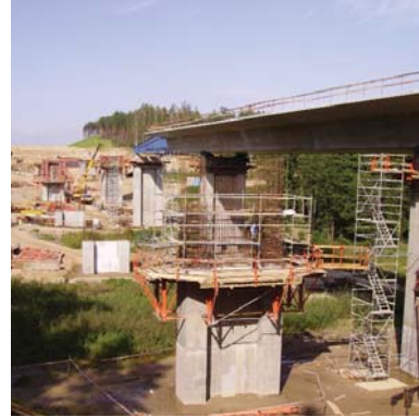
Bridge construction on the new A1 freeway in Poland
