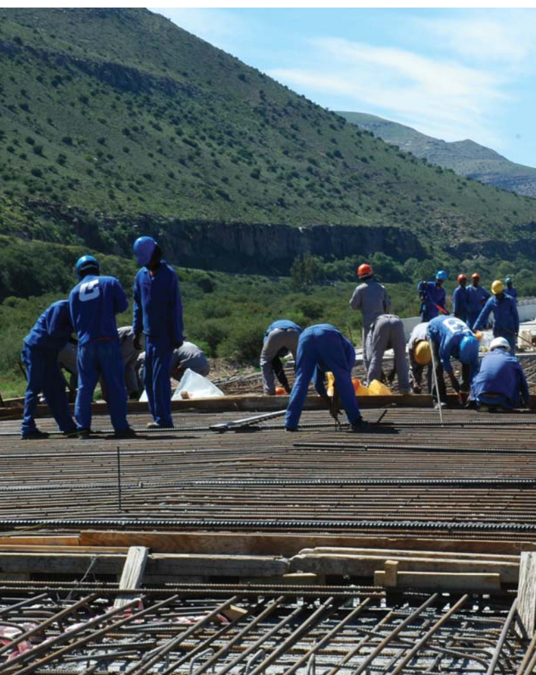
The Cradock road rehabilitation contract is the most recent to be carried out in joint venture with iLima
