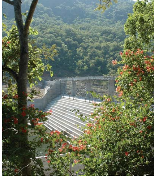
The Maguga dam regulating weir received a Fulton Commendation
