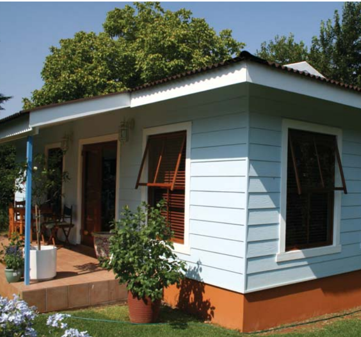
The prototype of a steel frame house uses Nutec products for cladding and internal finishes
