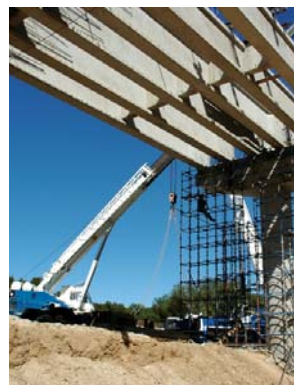
Bridge construction on the N10 south of Cradock in the Eastern Cape
