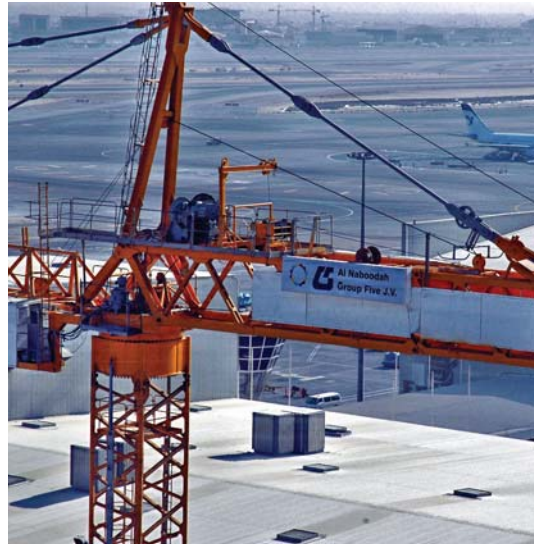
A crane at the CUC-6 contract at Dubai International Airport
