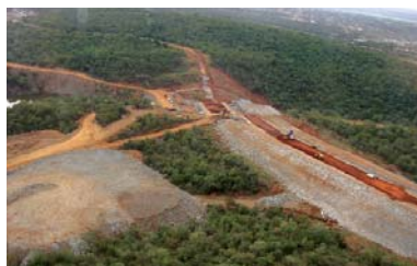
The Lusip dams contract in Swaziland will provide water to 2 500 subsistence farmers in the Big Bend area
