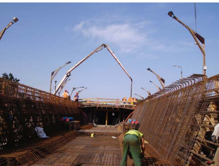
Bridge construction on the A1 in Poland
