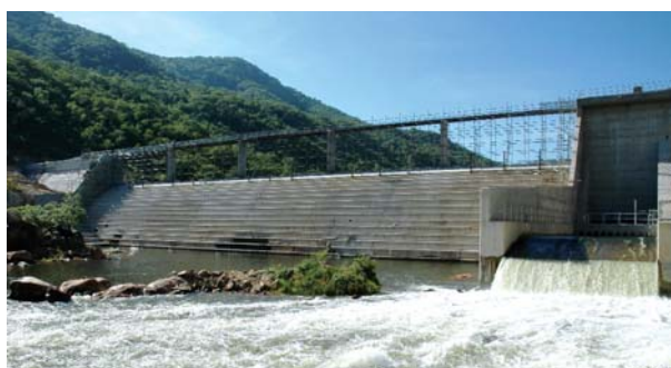
Construction of a regulating weir below the Maguga Dam in Swaziland
