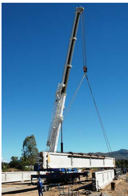
Lifting a pre-cast concrete beam for bridge construction on the Cradock to Tarkwa Bridge contract
