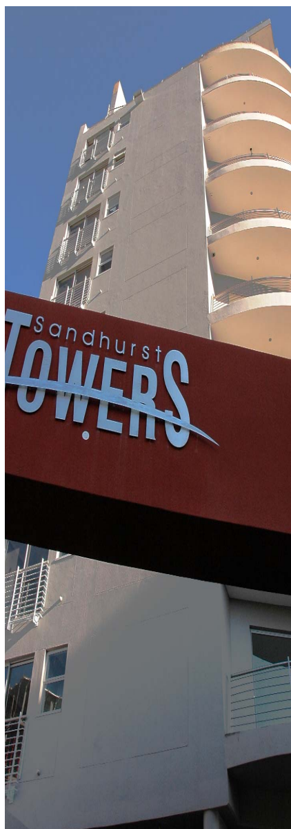
Sandhurst Towers was a key contract during the year
