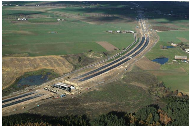
Road construction on the A1 in Poland
