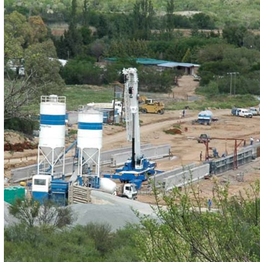
iLima Projects supplied concrete truck mixers on the Cradock Tarkwa bridge contract
