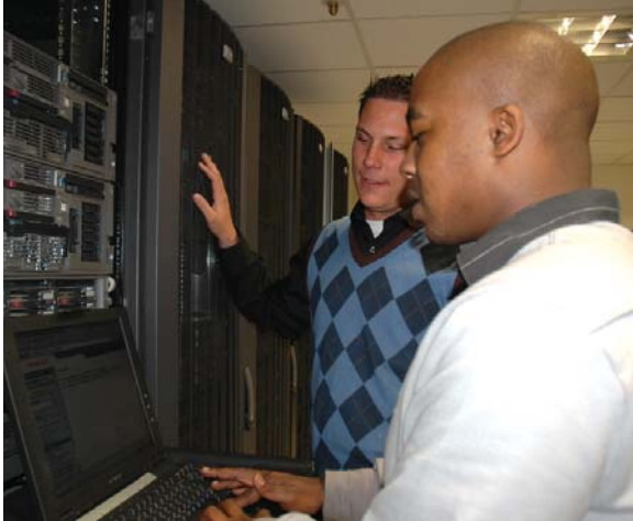
A new centralised server room has been installed
