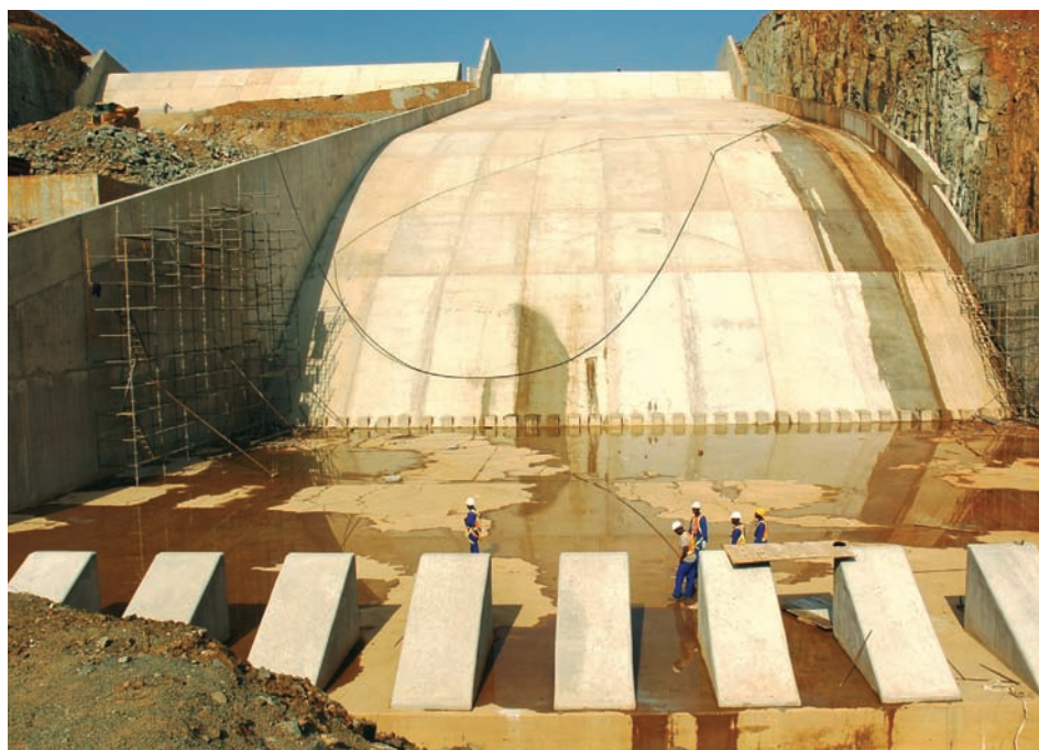
> The spillway at the LUSIP dams project in Swaziland
