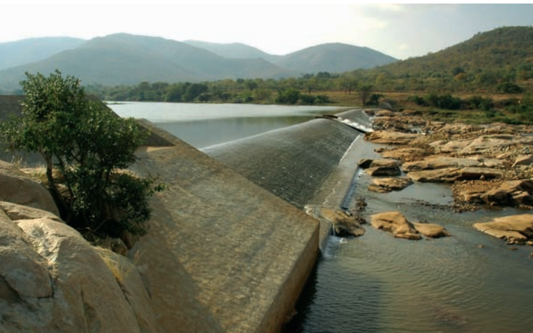
> A weir on the Lower Usuthu River in Swaziland maintains the flow of water to downstream users
