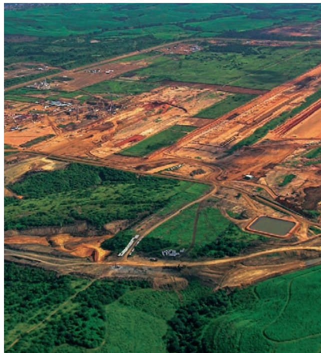
> New King Shaka International Airport under construction
