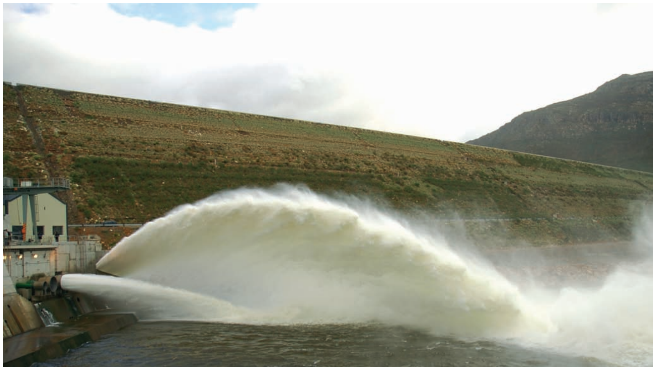
> Testing the flood gates at the recently-constructed Berg River Dam was executed in carefully timed increments to prevent flooding downstream
