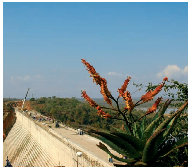
> Environmental controls at the LUSIP dams site in Swaziland have included the preservation of the surrounding flora
