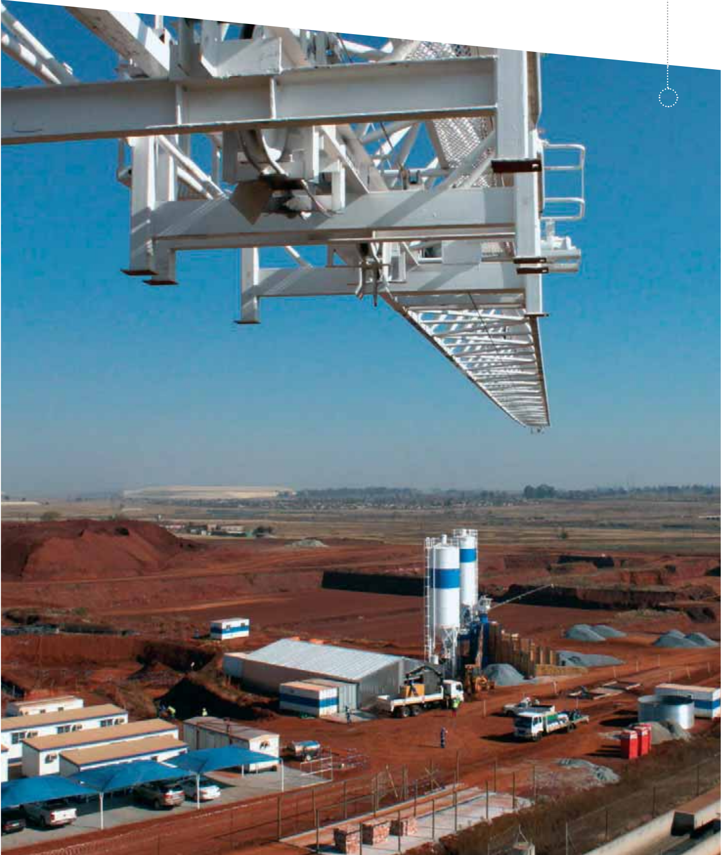
Welgedacht Water Care Works, Gauteng, South Africa
