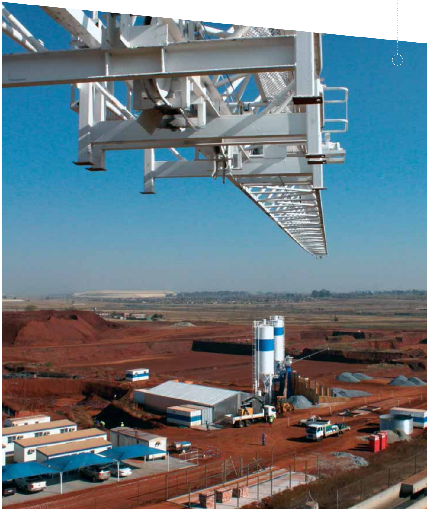
Welgedacht Water Care Works, Gauteng, South Africa
