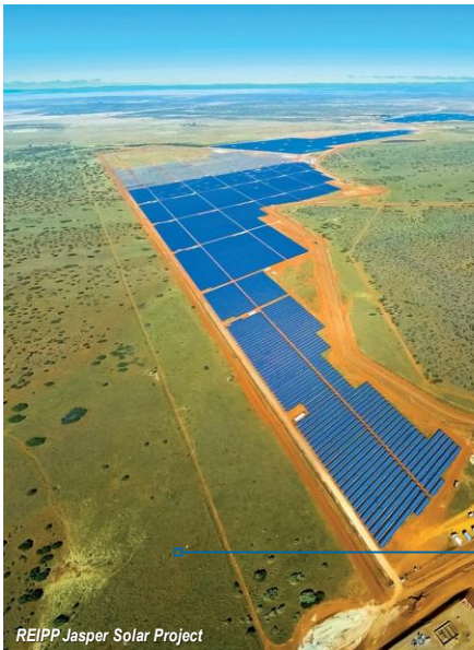
REIPP Jasper Solar Project
